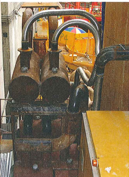
Central water scrubber to mitigate exhaust from air compressors and generators 中央水性隔氣鼓之作用是減少因操作空氣壓縮器及發電機時所產生之廢氣
