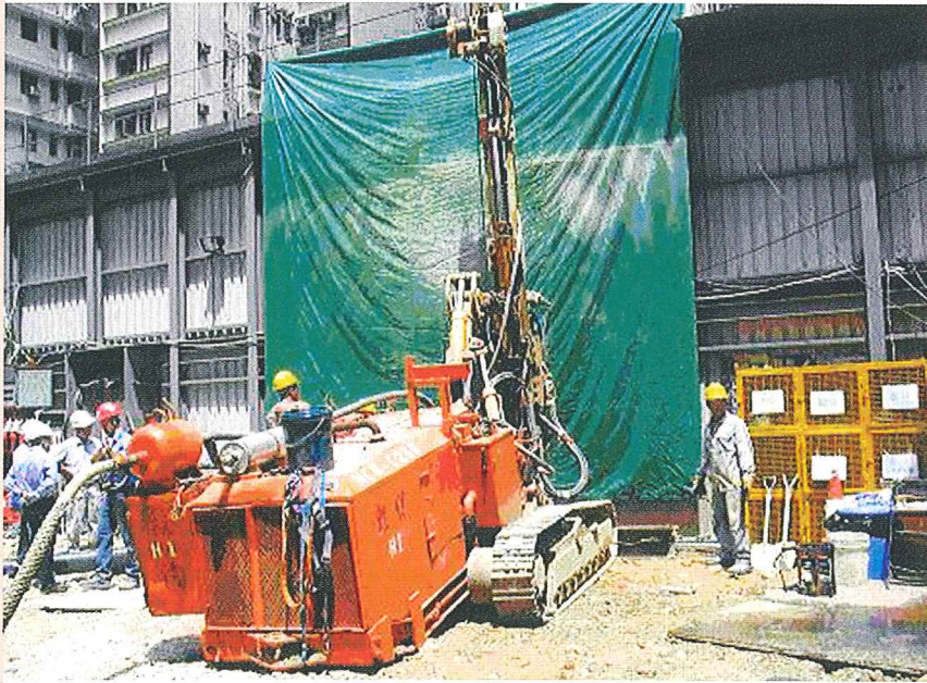
Dust screen for drilling works 為進行鑽孔工程而設之隔塵幕
